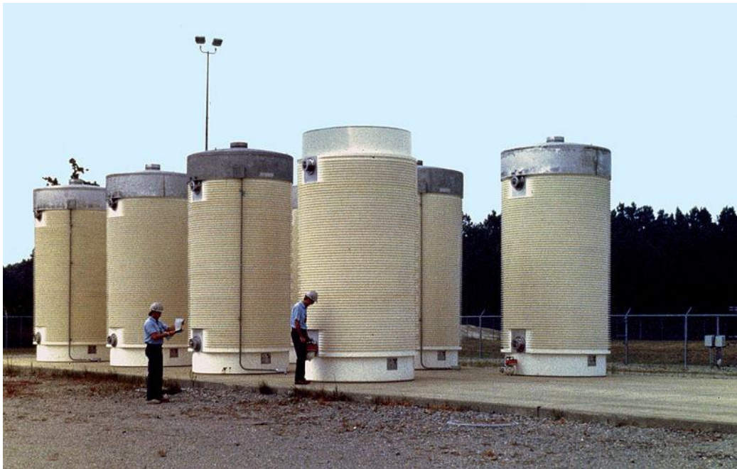
Onsite dry cask storage of used nuclear fuel (Image taken from Wikimedia Commons)
